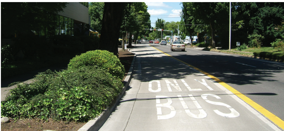
“Bus-only” lanes on LTD’s EmX bus rapid transit system (Photograph credit: CH2M)
